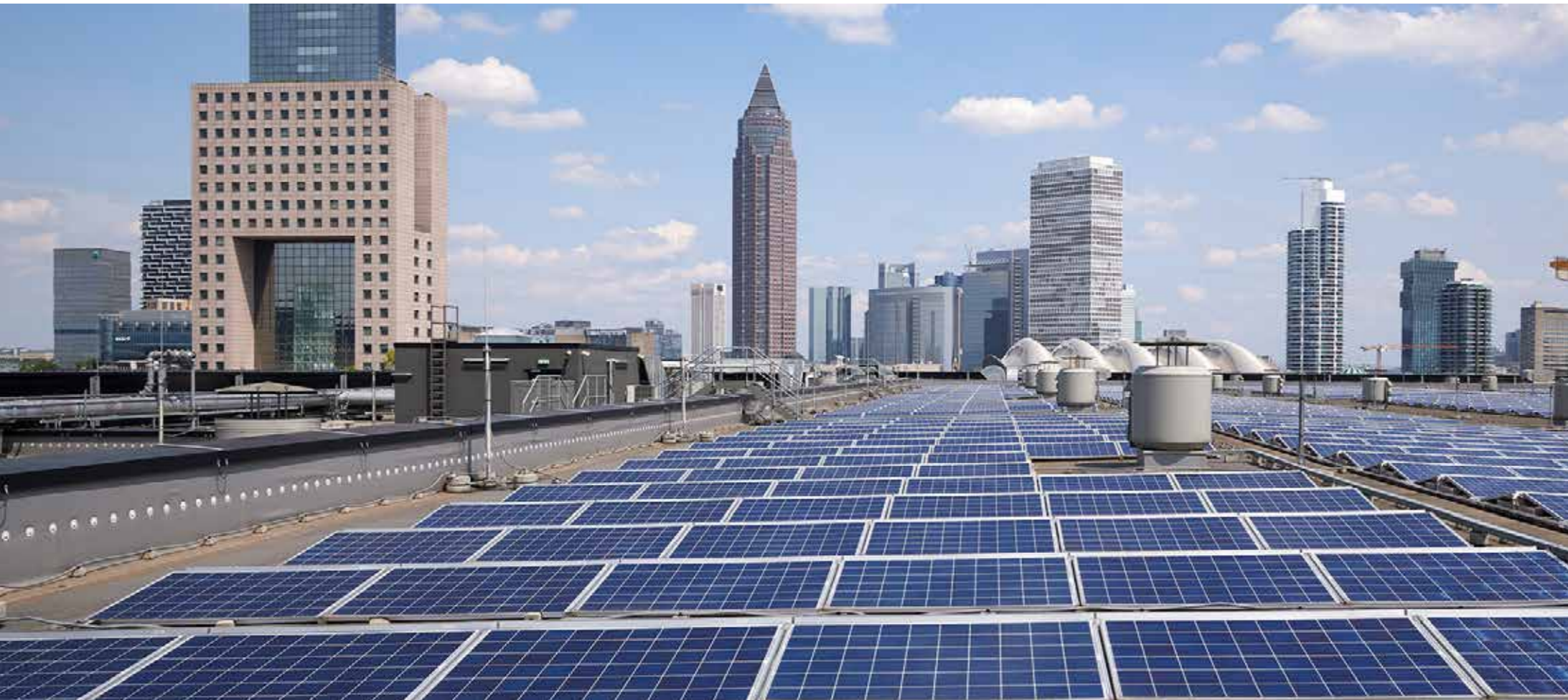
You need only take a look at the roof of the new Hall 12 to see that more sustainable use of natural resources has also long played a key role for Messe Frankfurt. ▲
